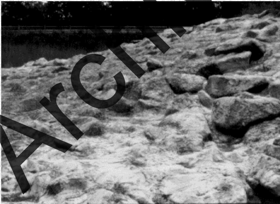
Figure 12. Grouted Riprap
