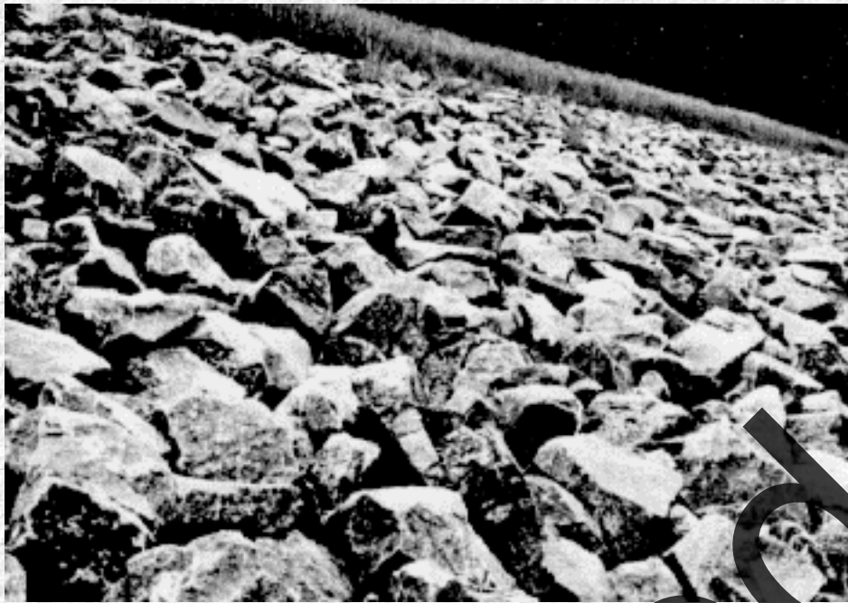
Figure 5. Dumped Rock Riprap
