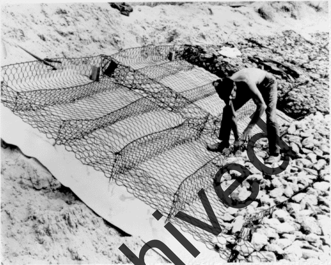
Figure 45. Rock and Wire Revetment Mattress Installation (courtesy, Maccaferri Gabions, Inc.)
