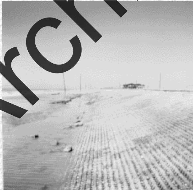
Figure 11. Pre-cast Concrete Block Mat
