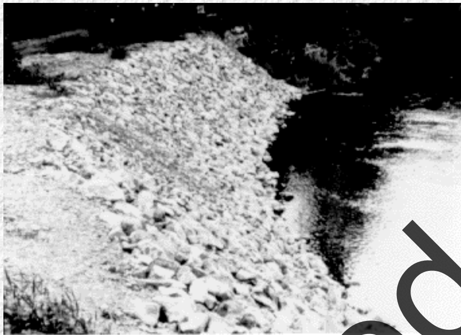
Figure 6. Hand-placed Riprap
