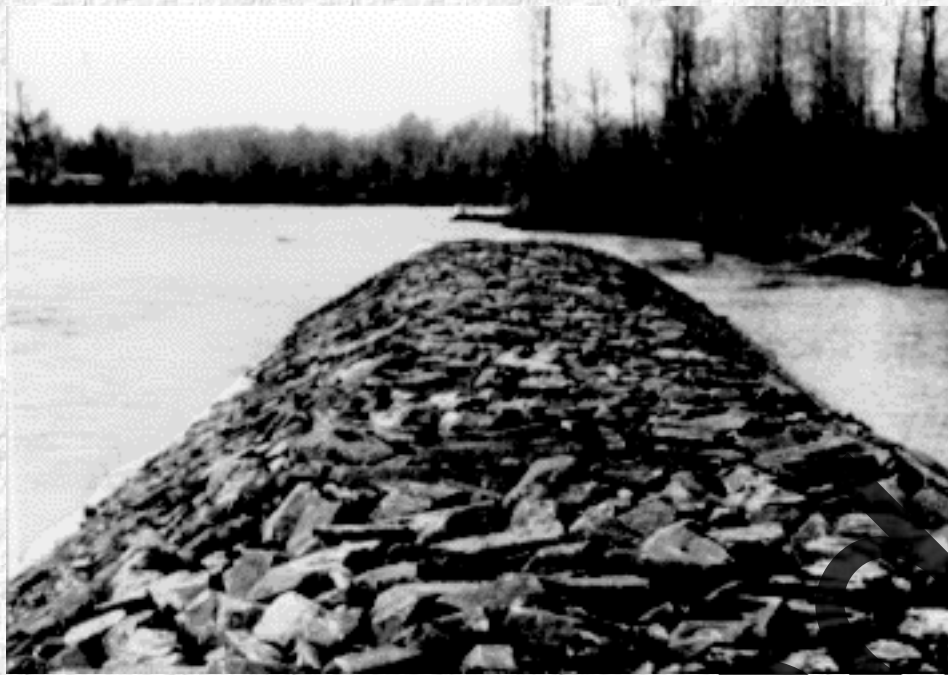
Figure 7. Plated or Keyed Riprap
