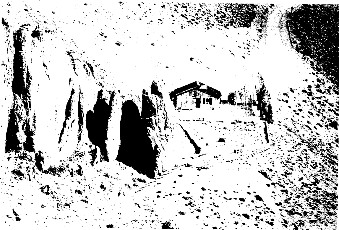
Figure 21: Detail of the end of the road, the visitor centre – warden housing and the beginning of the footpath. Fostering vegetation growth on the road cut is recommended.
